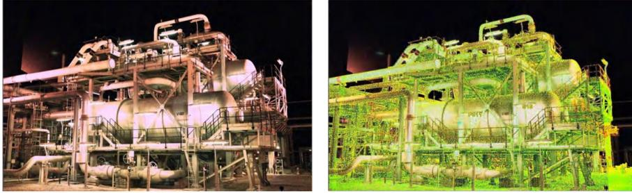
Figure 1: Part of a chemical plant and its scanned point clouds.
